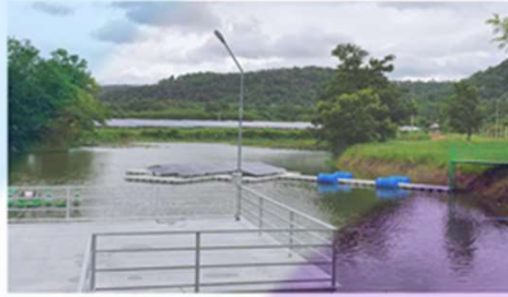
6KW floating system + 1MW ground system in Thailand
